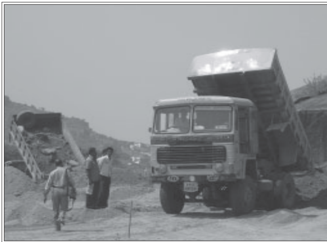
Full fledged work is being carried on at the site
